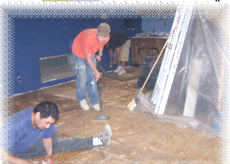
Floor prep in Cap'n Snow Assembly Room.
