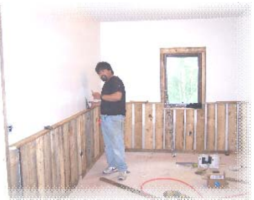
Wainscot being installed in VPSO office.
