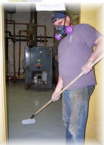
Todd Gage applying epoxy paint to resurfaced water plant floor.
